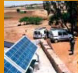
Photovoltaic (PV) energy, a power technology that uses solar cells to produce direct current, can be used to power equipment or to charge a battery.
